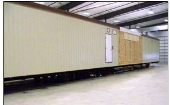
One of four building modules ready for shipping
