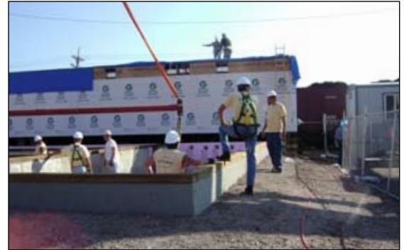
Preparing the foundation to receive modular units
