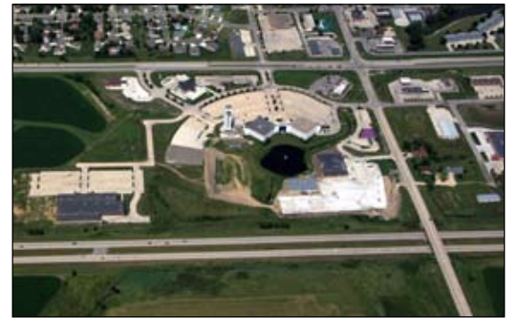
Aerial of project
